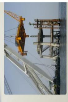
This Deck with the Equipment operates as a Wellhead Deck in which draws the gas from Hengam Field with a pressure, approximately 450 Bar and deliver this to Onshore Facilities to be treated with certain process.
