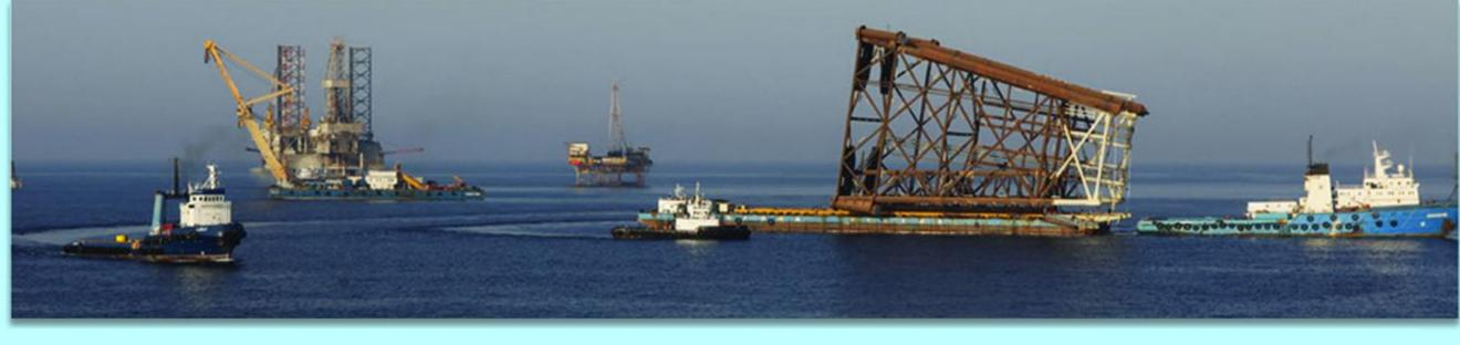
△ Design, construction, transportation, and installation of various offshore structures in different oil fields in the Persian Gulf, including the P4 jacket weighing 4,400 tons in the Reshdat oil field.
